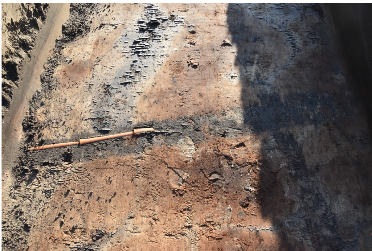
Fig. 2.14: Nutsleiding in sleuf 2.
