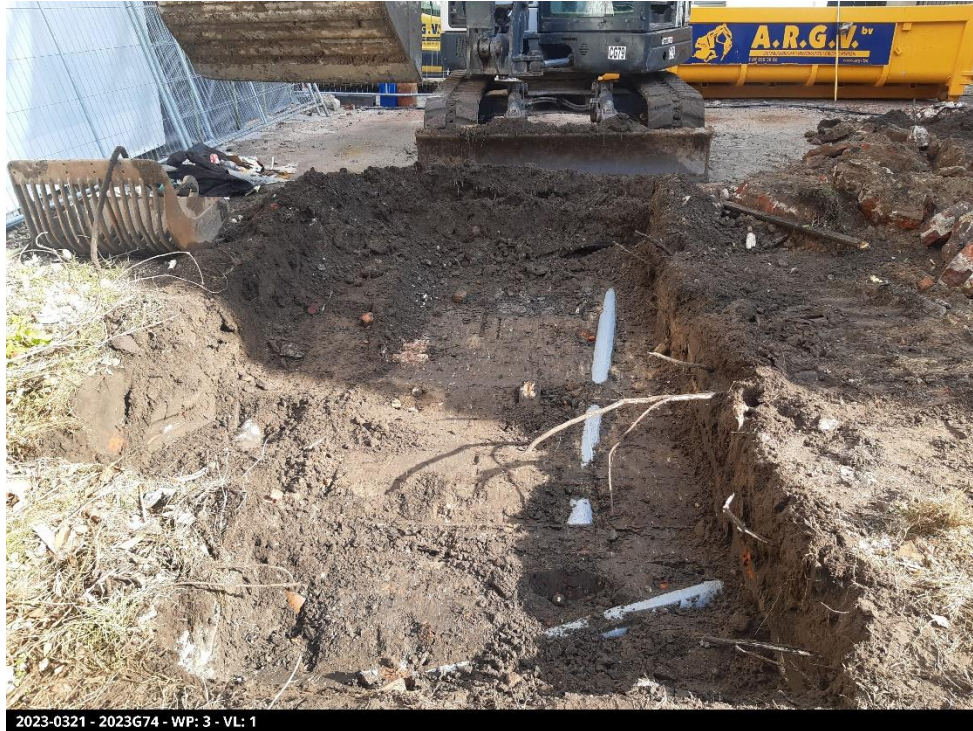
Figuur 28: Detailfoto werkput WP 3
