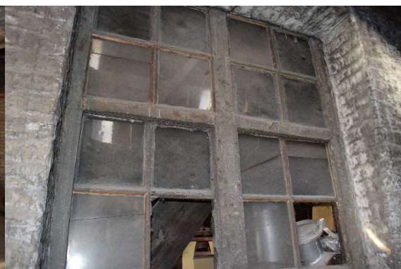
Afb. 586 M15h_R1.01: origineel 18 de of begin 19 de -eeuws houten raam
