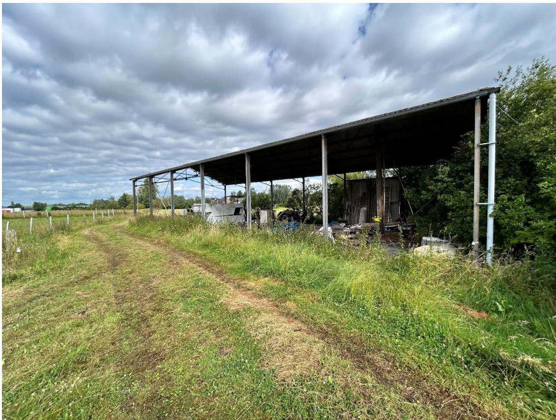
Figuur 7: Te slopen loods
