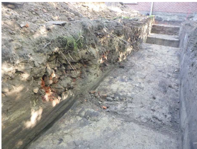
Figuur 16: Bouwpuin in de putwand in WP1
