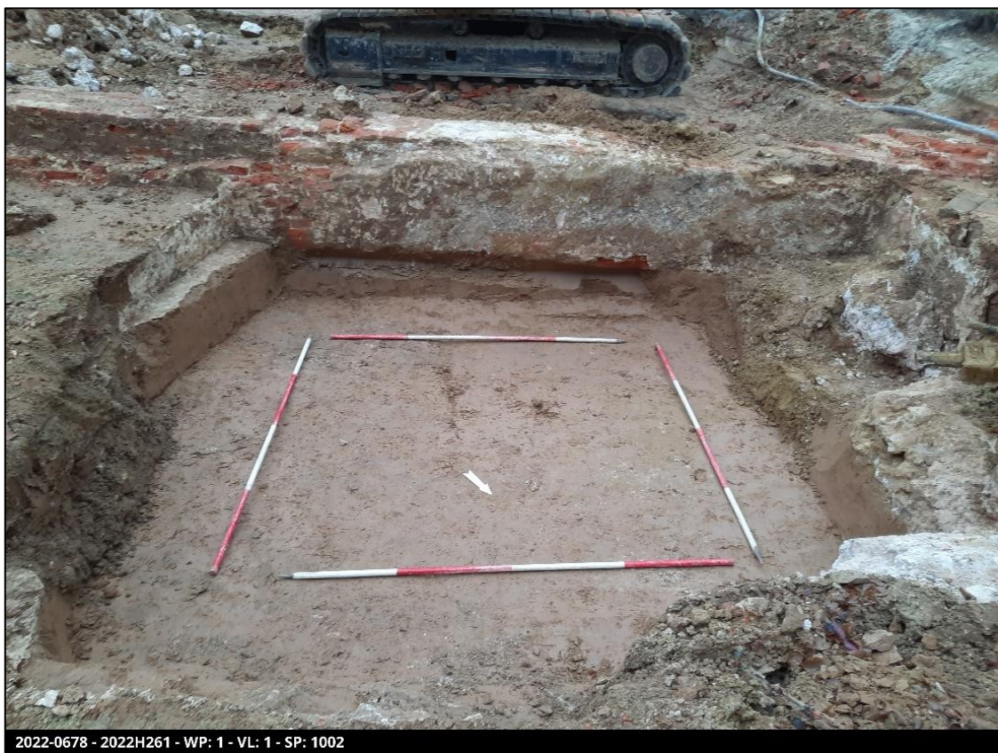
Figuur 10: Spoor 1002 in werkput 1
