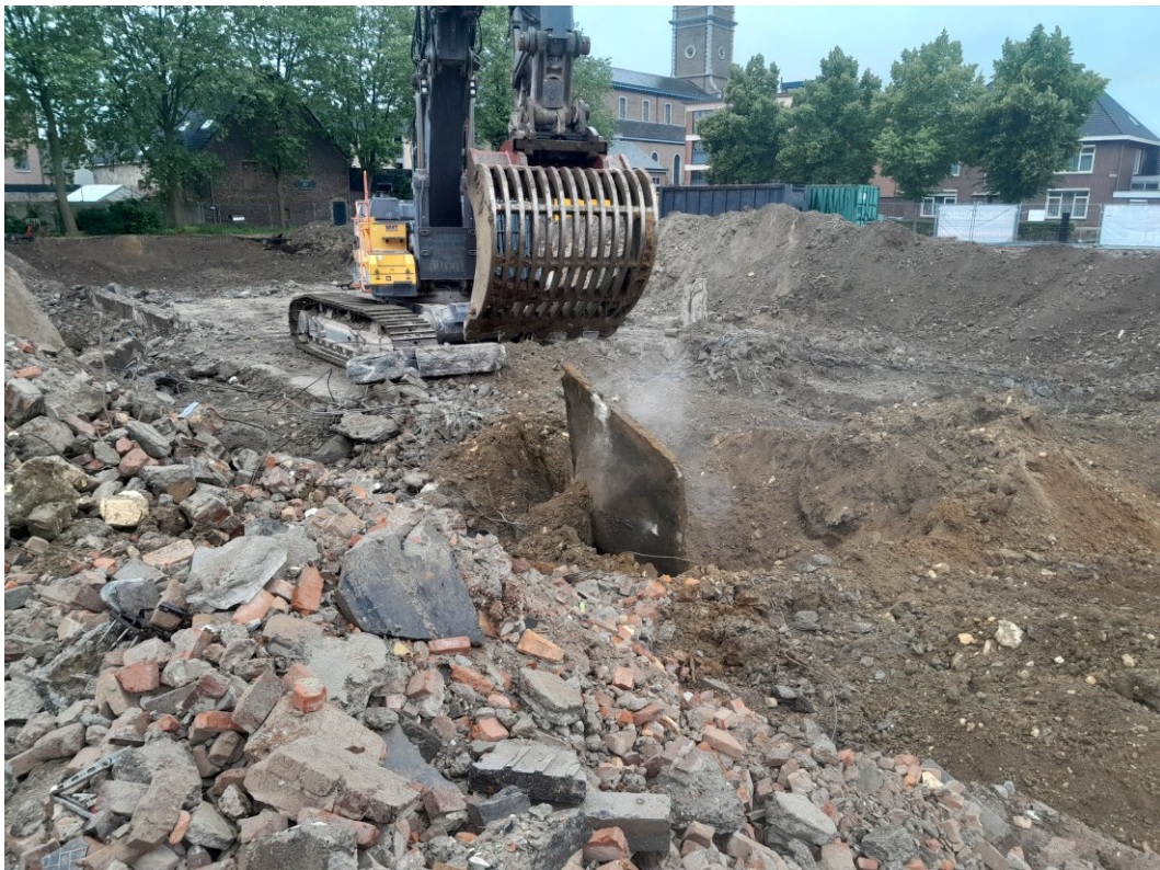
Figuur 30: foto 7: ontgraving funderingszool zone 5 (30/05, ABO nv)
